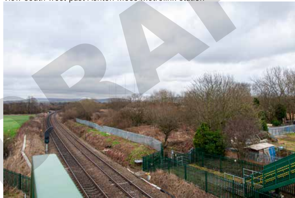
View of railway line to the north of the site, looking east from pedestrian railway bridge
